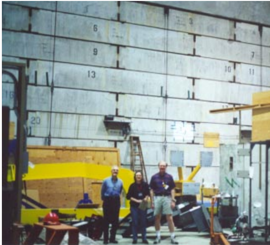
Figure 14-1: The area in the IR12 hall outside of the shielding wall where power supplies and klystrons will be located.
